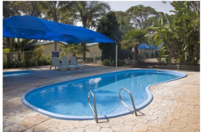
Changing pump operating times greatly reduced electricity consumption
