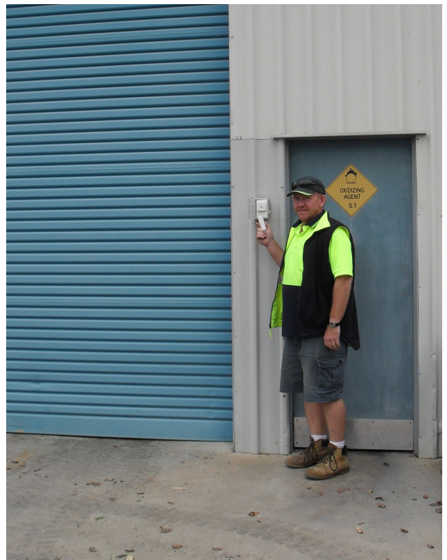
The use of hotel style key tags ensures that the high bay lighting in this storage shed gets turned off.
